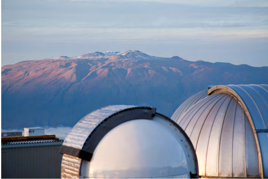
Figure 1. The 6 foot diameter VYSOS-5 dome (lower center) and the 12.5 foot diameter VYSOS-20 dome (right) at the Mauna Loa Observatory located at 11,135 feet above sea level on the North slope of Mauna Loa on the Big Island of Hawaii. The domes of observatories on Mauna Kea can be seen on the peak in the background.
