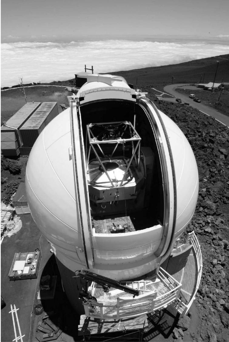
**Figure 1.** The prototype Pan-STARRS telescope installed near the top of Haleakala, Island of Maui, Hawaii. All the optics are in place, the dome is operational and first light has already occurred. Installation and testing of the OTA camera (near the center of the primary mirror) is the next step.
